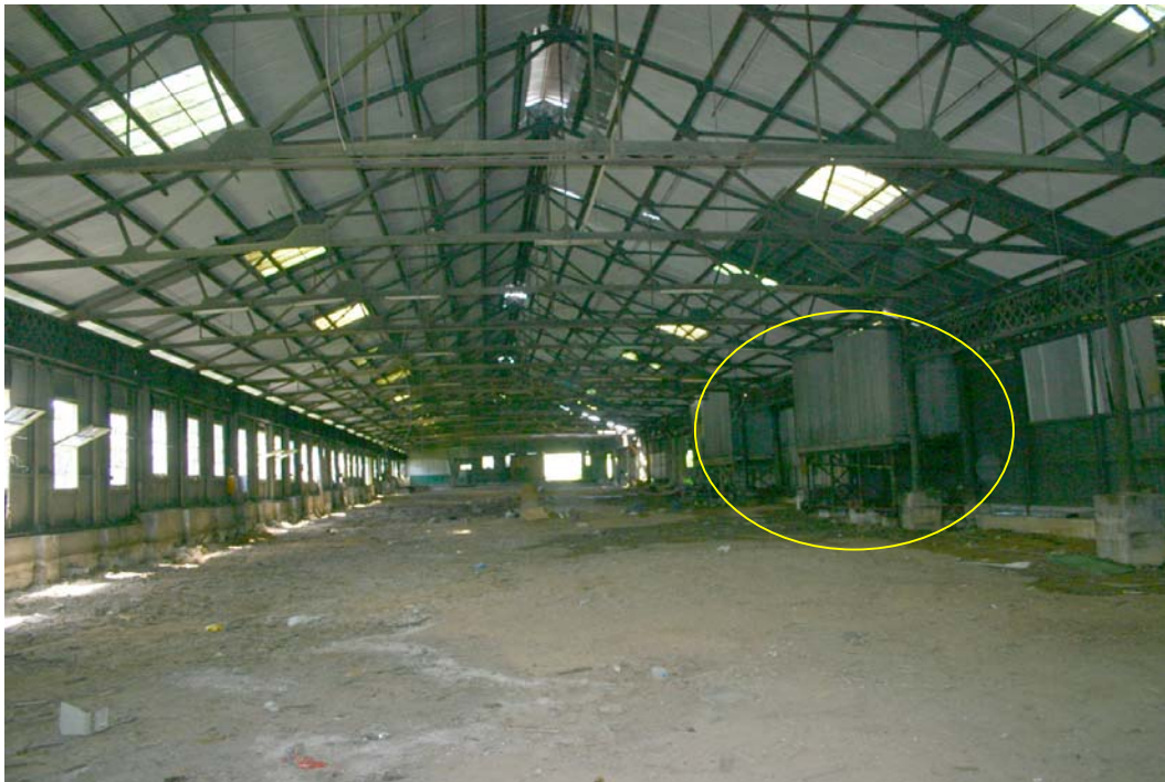
Figure 61. Interior of bay 2 of the Tarpaulin Factory, Columns are arrayed along each wall section. A toilet and shower complex (yellow) is set into the centre of the building. January 2005
