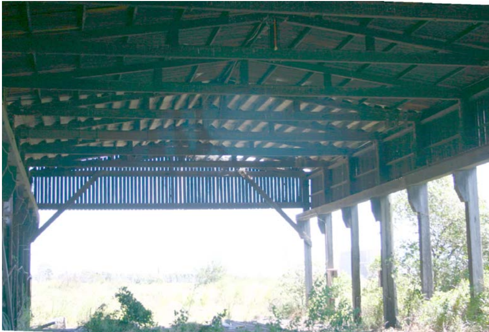
Figure 39. The internal structure of the Transhipment shed & wagon repair workshop showing the palings enclosing the gable ends and the bolted braced frame construction.
