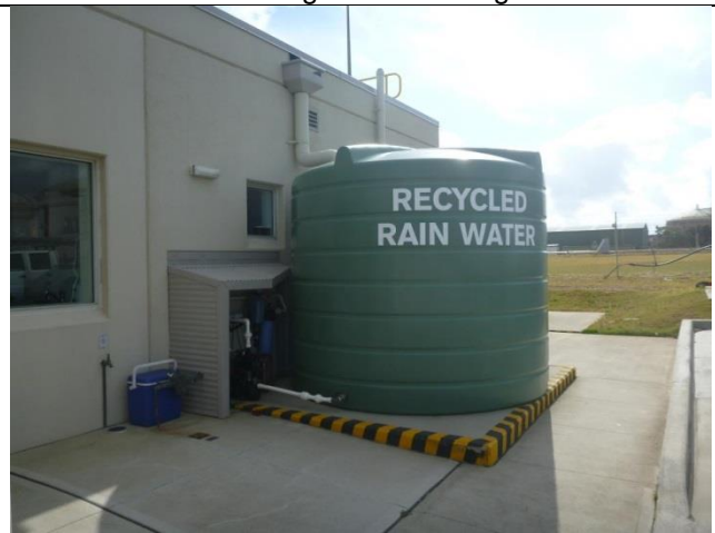
Photo: 4: Rainwater tanks for non-potable use in the operations building
