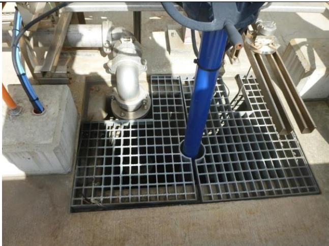
Photo: 9: Liquids spilt on the deck would flow to this low point – would be pumped back to the spill containment tank on shore
