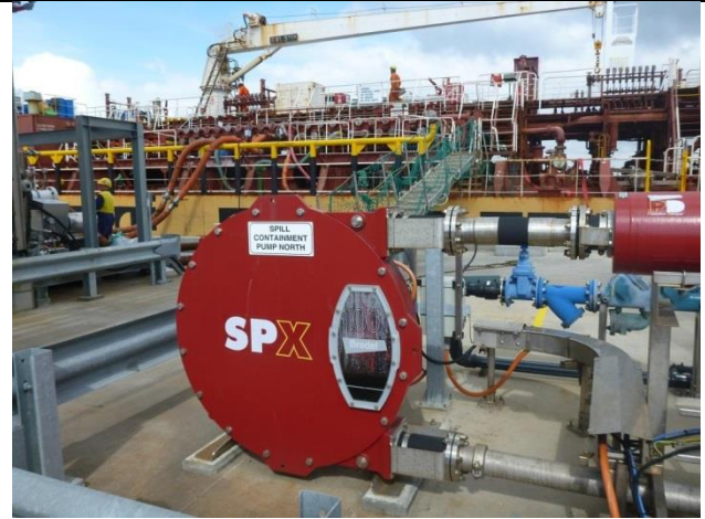
Photo: 8: Spill Containment Pump (north) on working platform. Would be used to pump spilled liquids back to the spill containment tank on shore. (regularly tested)
