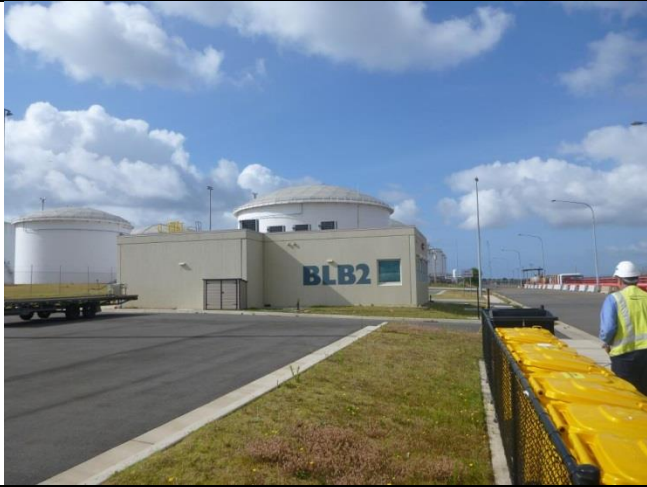
Photo: 1: View of the Operations building and car park
