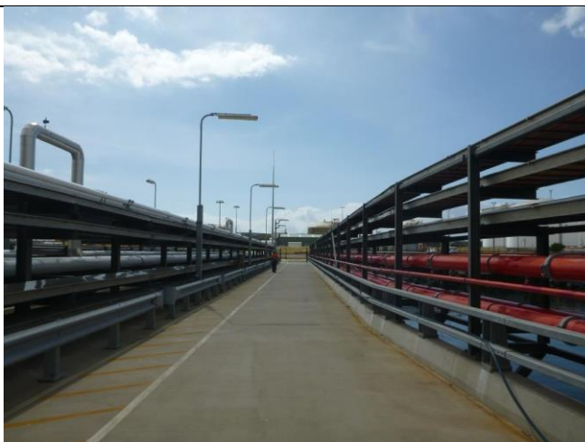
Photo: 11: View of access roadway from shore to working platform
