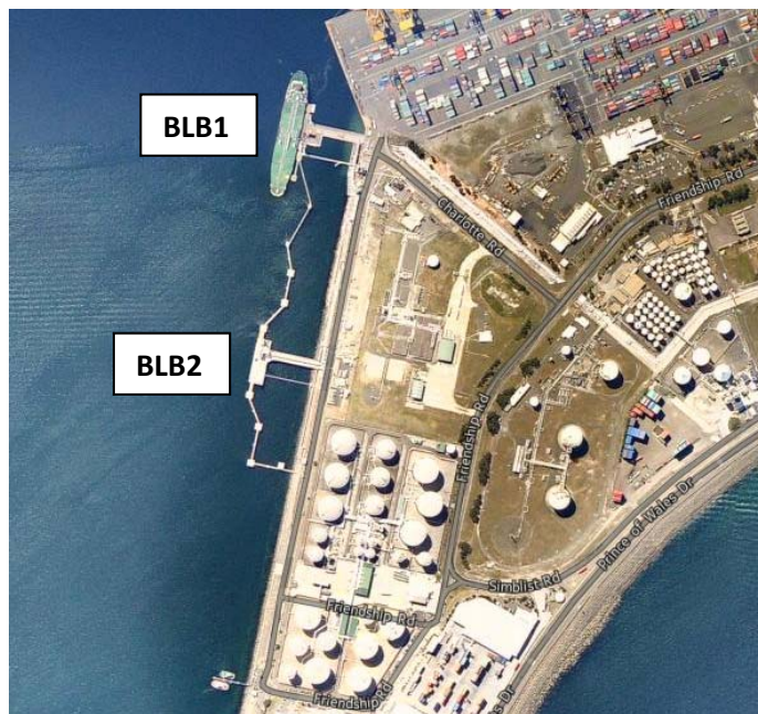
Figure 1: Location of BLB2 infrastructure
