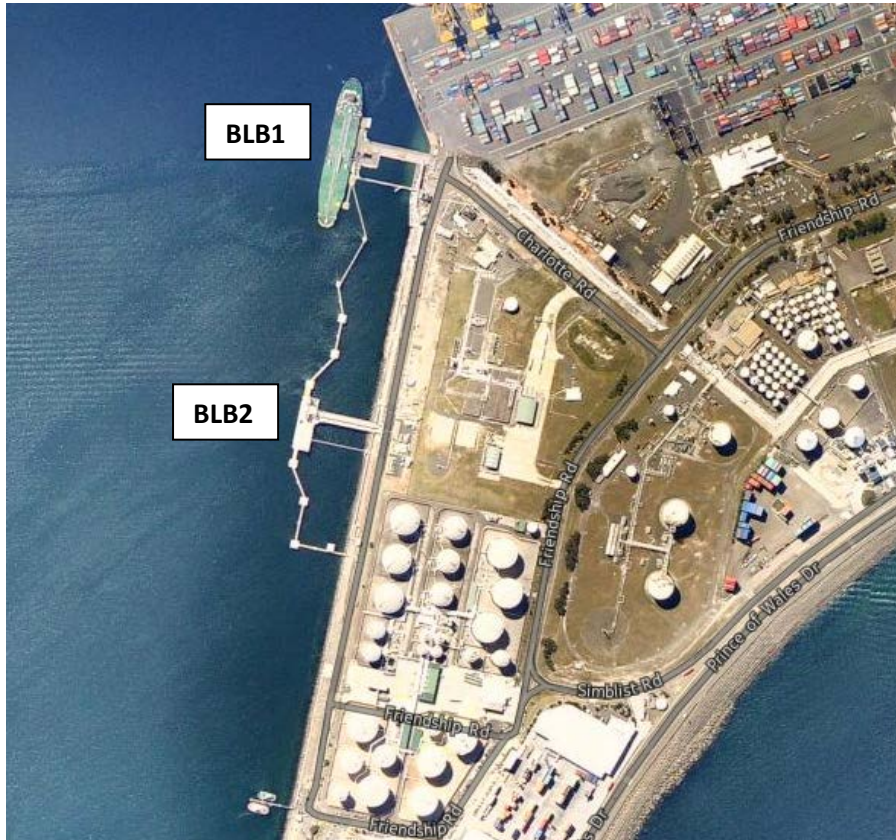
Figure 1: Location of BLB2 infrastructure
