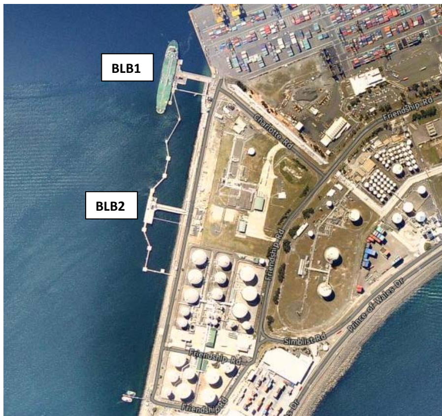
Figure 1: Location of BLB2 infrastructure
