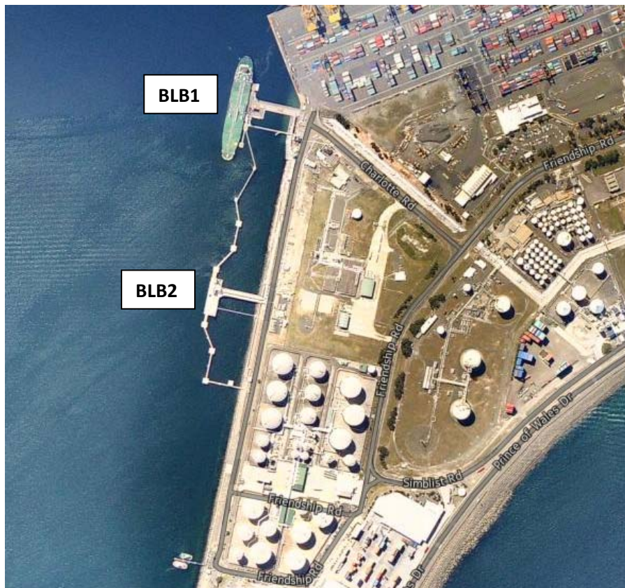
Figure 1: Location of BLB2 infrastructure
