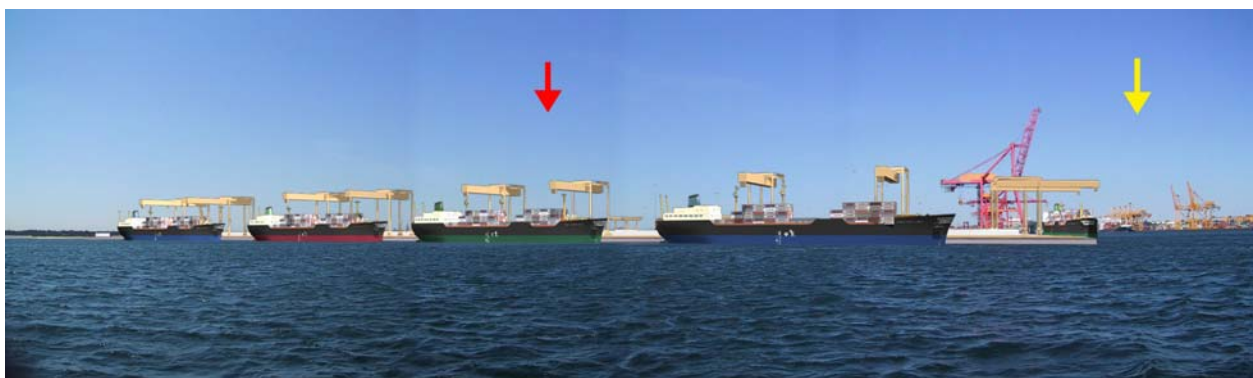
View of the proposed Port Botany Expansion. The yellow arrow indicates the location of the existing Port Botany. The red arrow indicates the location of the proposed Port Botany Expansion.
