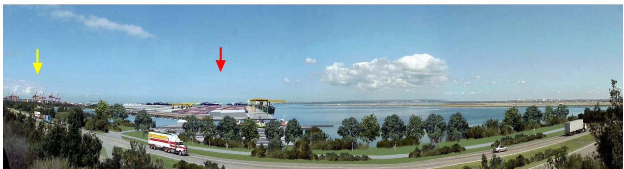
View of proposed Port Botany Expansion, Sir Joseph Banks Park. The yellow arrow indicates the location of the existing container terminals at Port Botany. The red arrow indicates the location of the proposed Port Botany Expansion.
