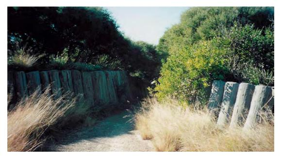
Plate 4: Substantial timbers have been used as a retaining wall at one of the entrance ways to the Sir Joseph Banks Park.
