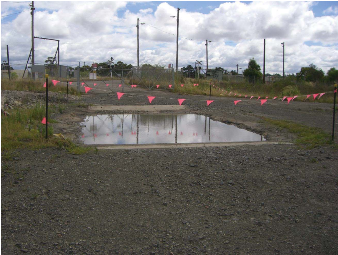
Figure 3 Wheel wash facility at ILC Site
