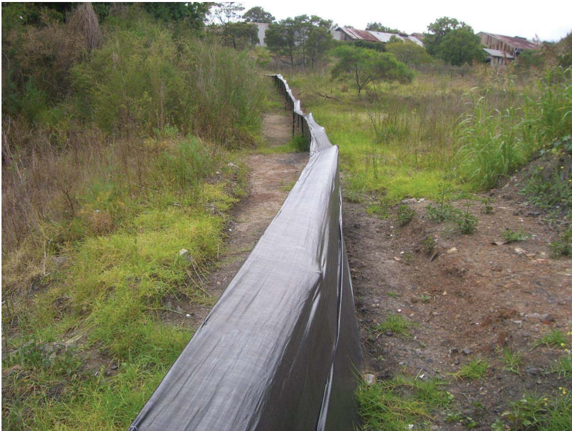
Figure 2 Frog habitat protection fencing near Coxs Creek
