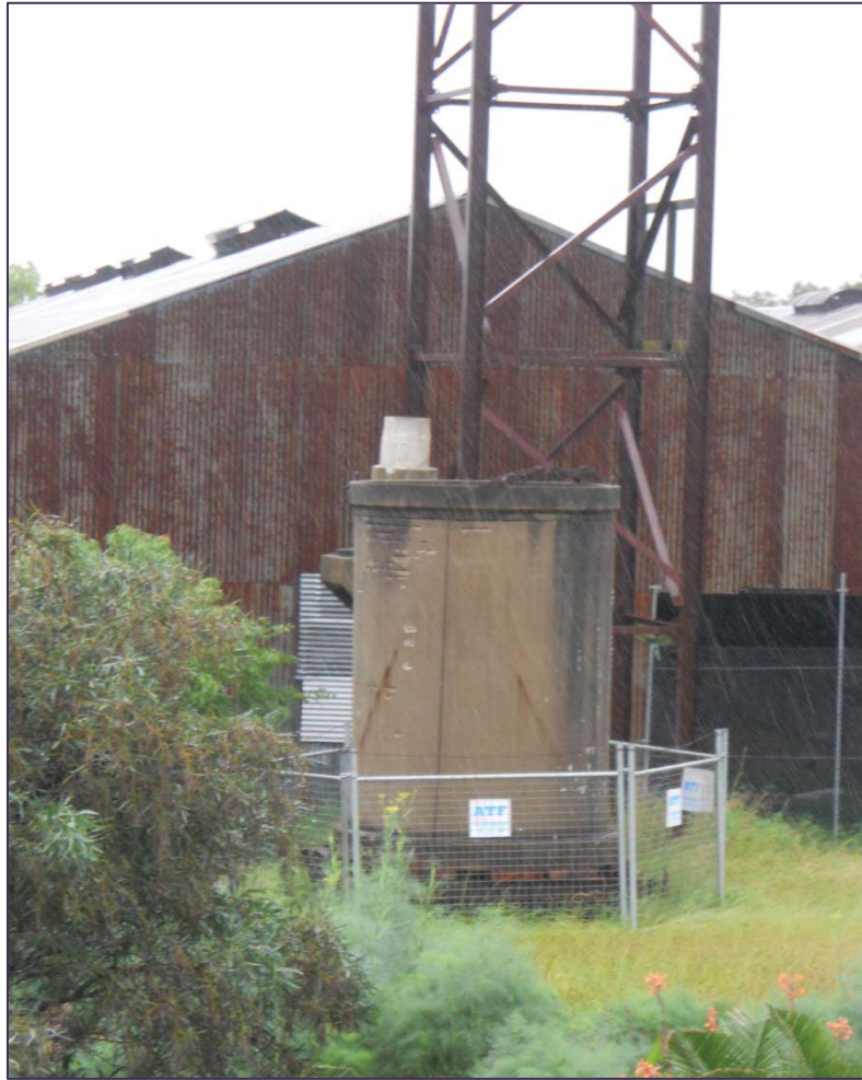
Plate 2: Tarpaulin Shed (background) with Pillar Water Tank (foreground)
