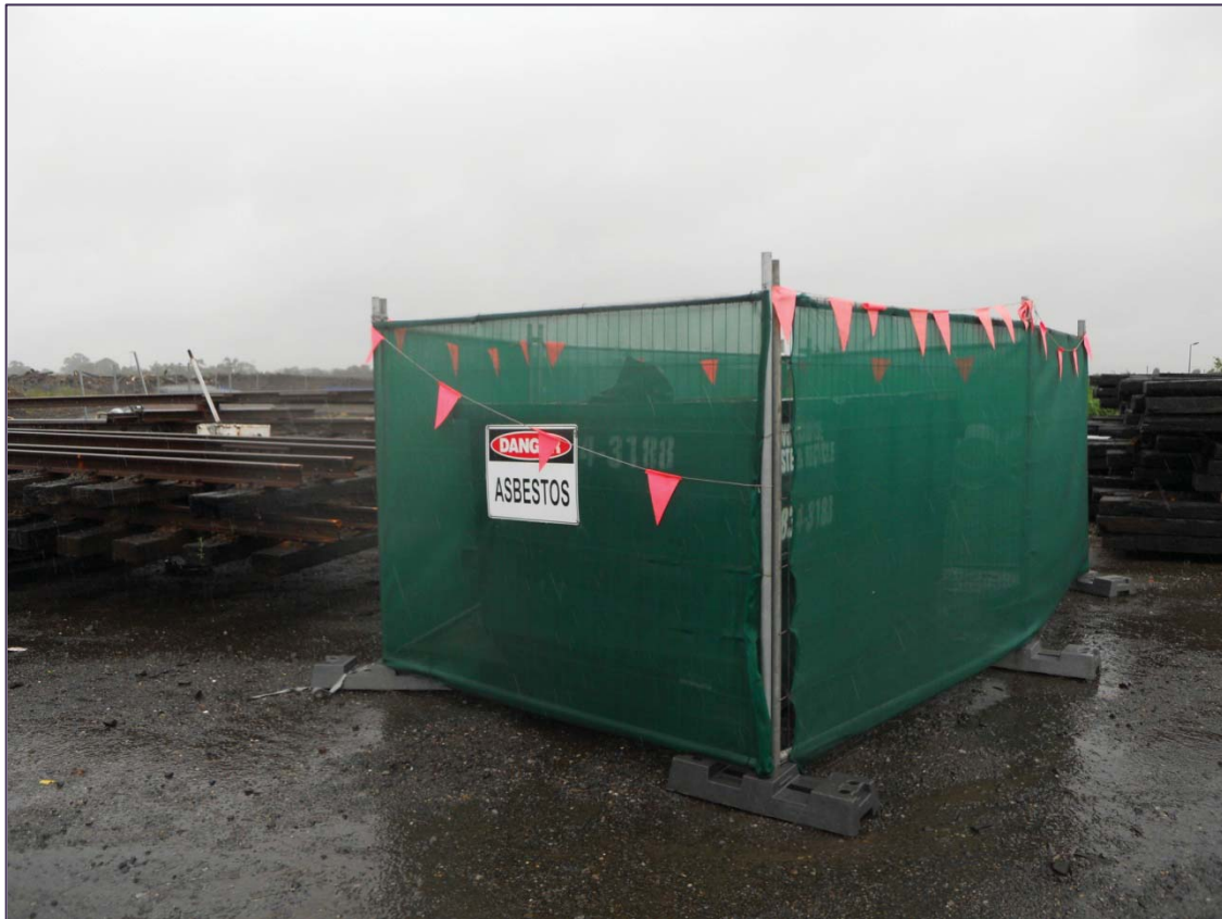
Plate 3: Asbestos storage skip in protective enclosure
