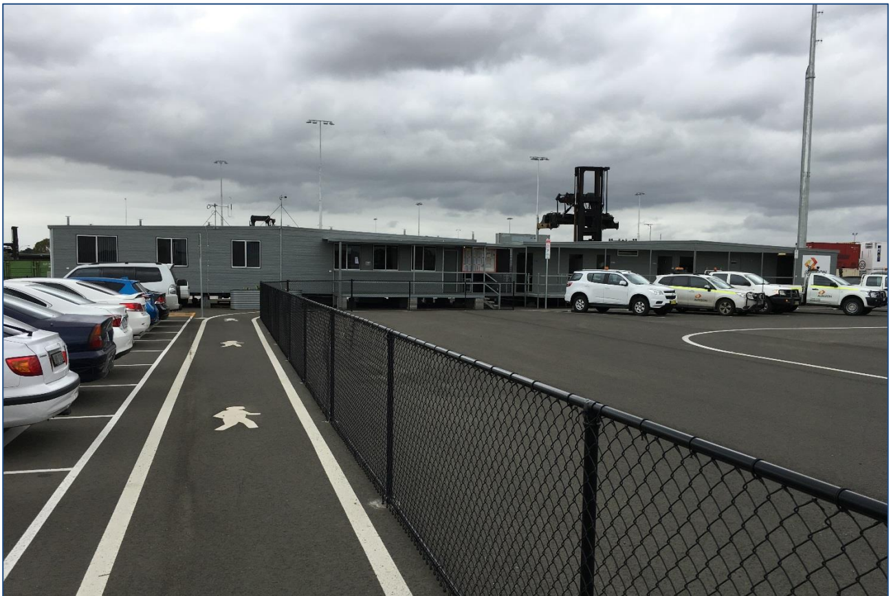
Figure 5 - Existing Intermodal Terminal Administration Building (source: NSW Ports)
