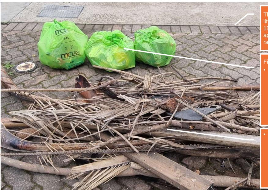
The first clean out of the litter trap was completed 15 August 2024 after approximately 30 mm of rain over 35 days.
