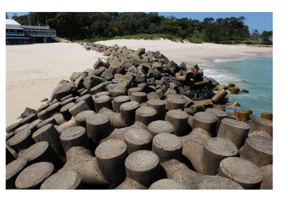
The groyne was strongly constructed. From high water mark it is shielded by tightly packed and interlocking <u>dolosse</u>.
