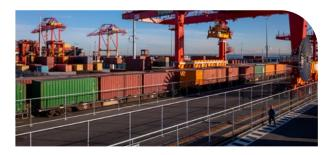
The only port in Australia with on-dock freight rail at every container terminal, which increases efficiency and removes the need for double handling by trucks.
