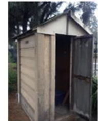
3. Precast Concrete Hut 2
