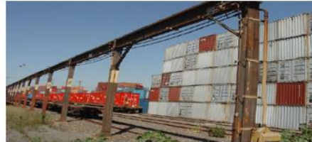
5. The Electric Overhead Travelling Crane
