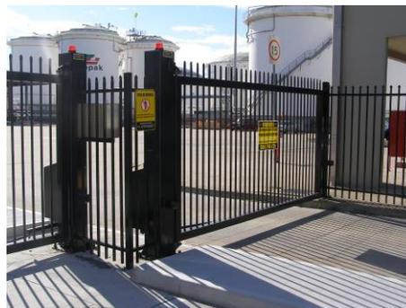
**Figure 6** - Security chain wire gates with 3-strand barbed wire (left) and security palisade gates and spiked caps
