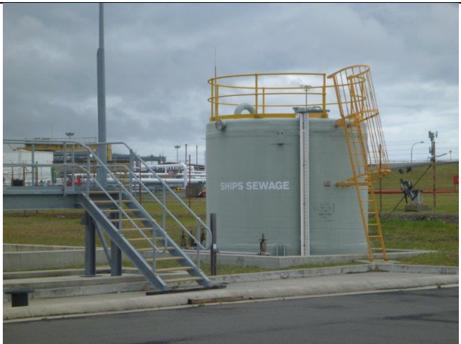
Photo: 9: Sewage tank installed to accept ships sewage. The tank has not been used to date and remains empty.
