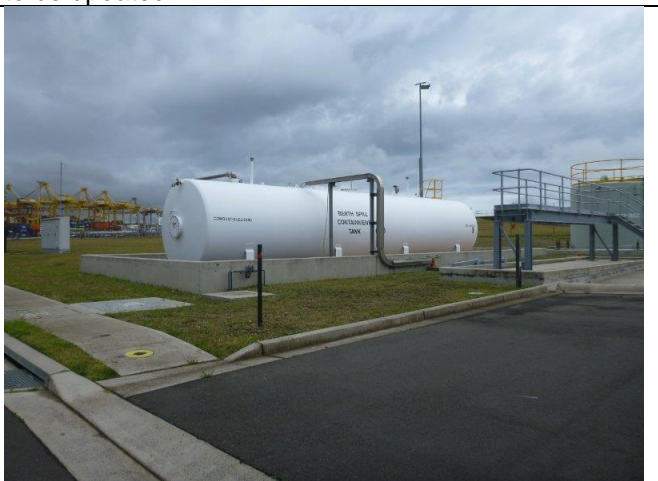
Photo: 5: Berth spill containment tank (empty) – fully bunded. Would be used in case of spill at the berth and on site
