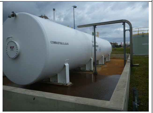
Photo: 6: View showing spill containment tank with bund.
