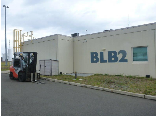
Photo: 1: View of the Operations building and car park. Forklifts used to transport various goods and drums
