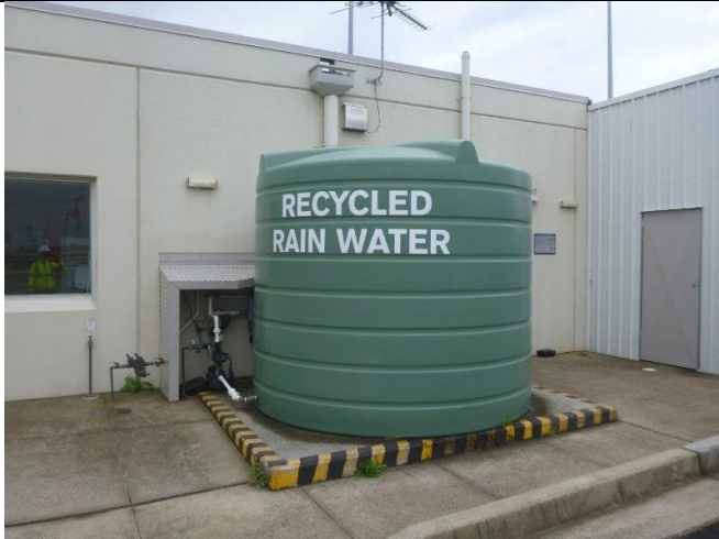
Photo: 7: Recycled rainwater tank u
