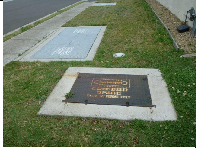
Photo: 8: Gross Pollutant trap and oil water separators installed underground. Cleaned out in 2016.
