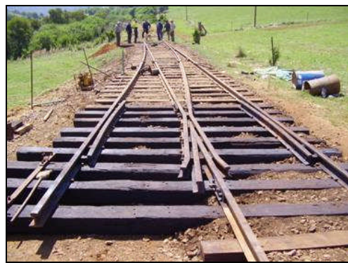
Reclaimed track work re-installed on site at Dorrigo.
