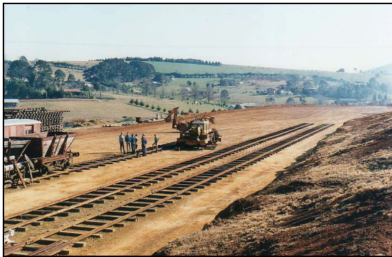
Reclaimed track work re-installed on site at Dorrigo.
