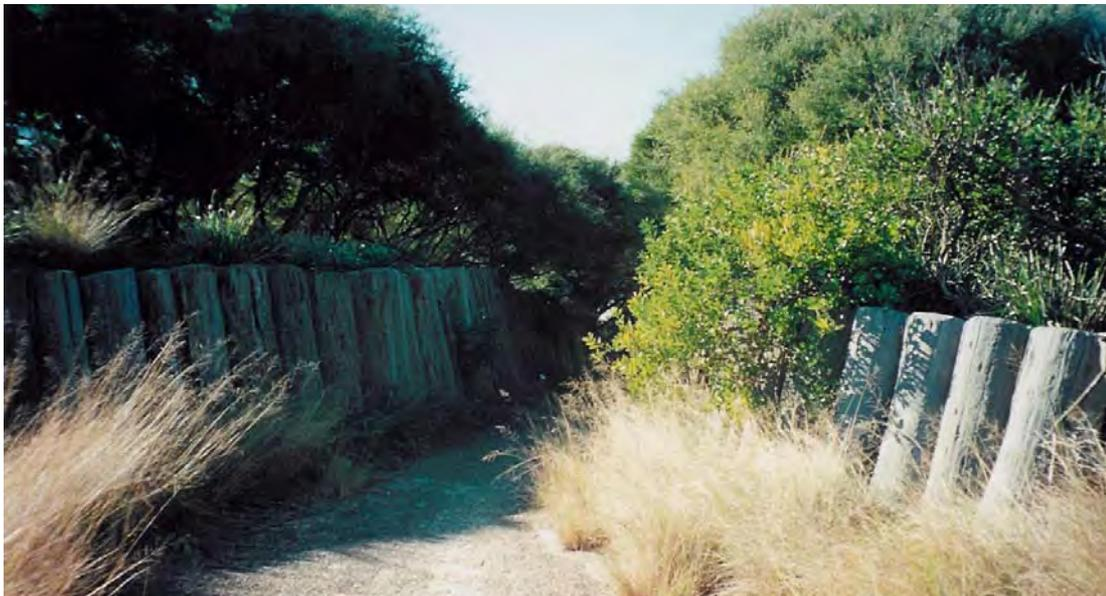
Plate 4: Substantial timbers have been used as a retaining wall at one of the entrance ways to the Sir Joseph Banks Park.
